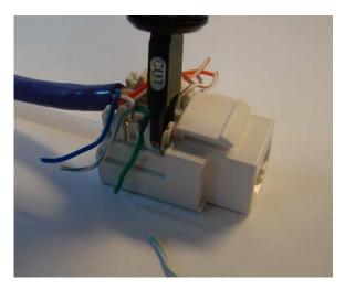
**Step 3.** Place the blade of your punch down tool over each wire and press down firmly until you hear the tool snap. If you are using a cut blade, make sure the cutting tip is on the outside of the connector. The cutting tip will trim away the excess wire automatically. Do this for all 8 wires.
