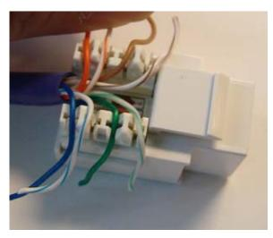
**Step 2.** Untwist and splay out the wires and sort them through the appropriate slots on the connector. Follow the color coding diagram on the inside of the connector for the proper wiring standard you wish to use.
